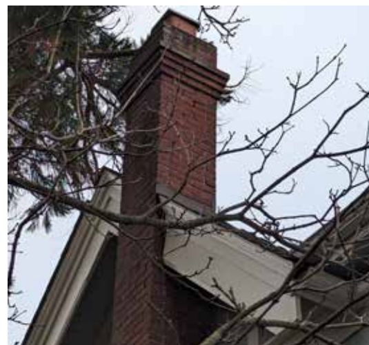
Top and Bottom: Red brick chimney with grey mortar and corbelled top associated with the 1921 addition.
