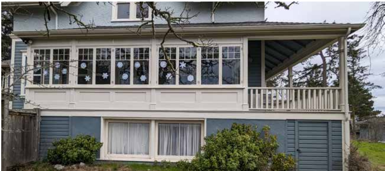
Top Left and Right: Second floor balcony on east elevation. Above: Enclosed portion of wrap around verandah with pairs of casement windows and wood panels below.
