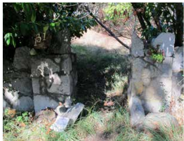
Top: Stone wall with crenulated cap on square gatepost to west of driveway access from Brighton Avenue terminus.
