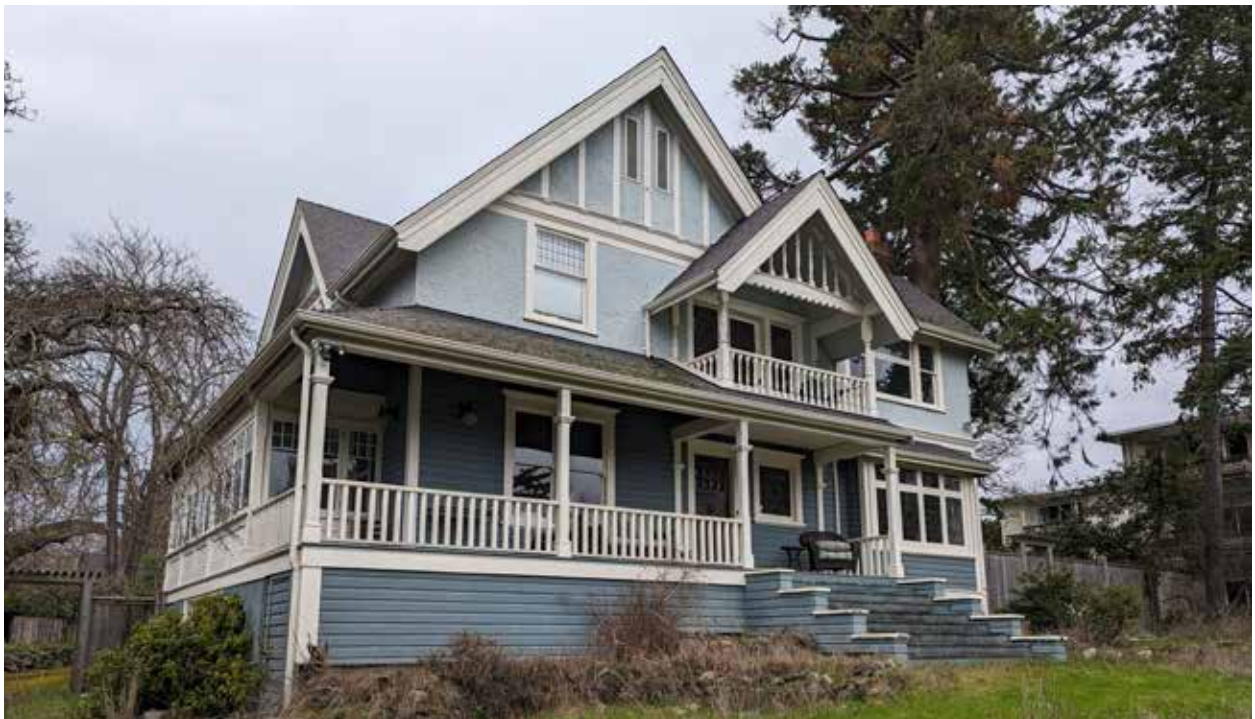
Below: Exterior stucco and wood cladding and wood detailing of east and south elevations.
