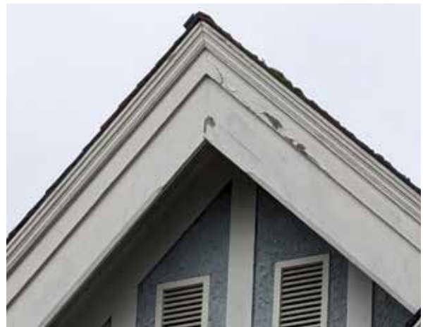
Top: Wood rot at fascia on rear addition. Middle and Bottom: Photos of representative paint failure.
