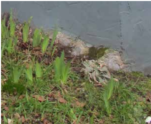
Above: Stone foundation with later applied parging at south-west corner of c.1896 portion of residence.
