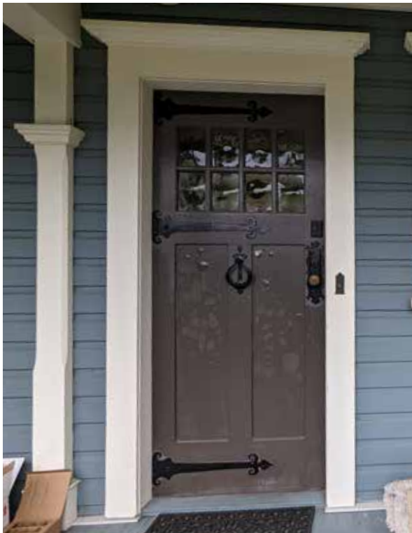
Above: Victorian period multi-panel wood door with blown glass insets, iron straps and original hardware.
