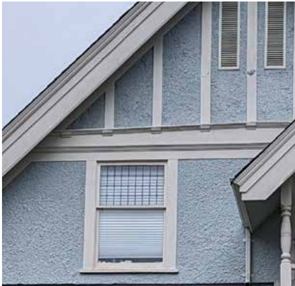
Above: Stucco of second floor and gable of east elevation. Top Right: Close up of texture finish of cement stucco.
