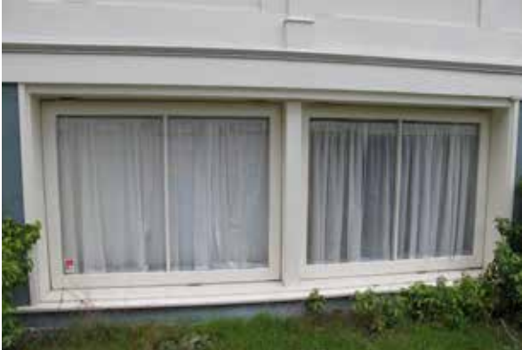
Above: Basement level wood awning style windows to be rehabilitated to suit new use and code requirements.
