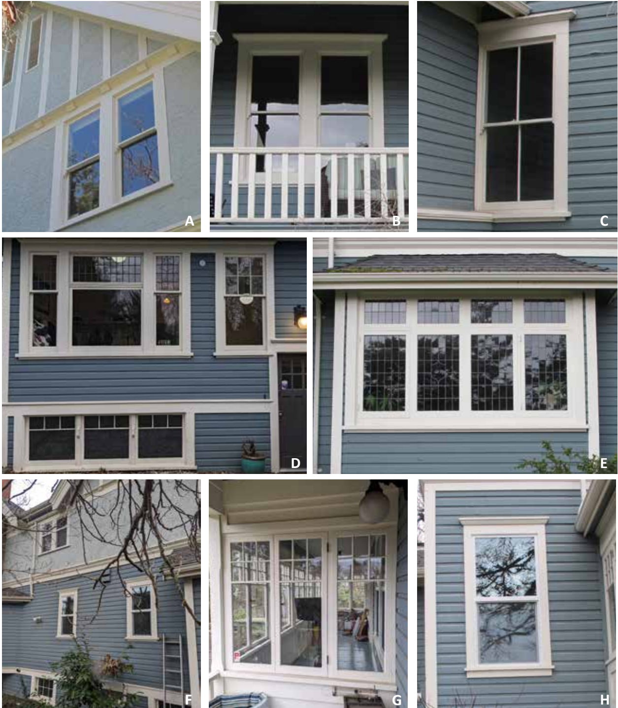
A- Double assembly, one-over-one hung windows; B- Double assembly, one-over-one hung windows with crown moulding; C- Single assembly two-over-two hung window; D- Single assembly six-over-one hung window, hung window with multi-lite leaded glass upper and single-lite lower sashes on either side of fixed single-lite window with multi-lite leaded glass transom; E- Bank leaded glass fixed and casement windows with multi-lite leaded glass transoms; F- Windows of north elevation with modern interventions; G- Multi-lite fixed and casement windows of enclosed verandah; H- Non-original window opening with modern window and casing similar to original window casings.
